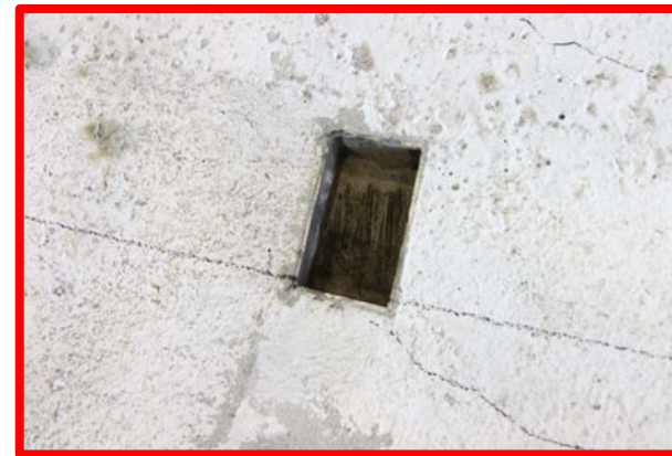
Notch at middle support top to flame cut the strands
